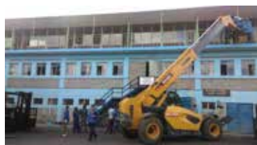
XCMG telescopic handlers help constructions of a factory building in Ethiopia
